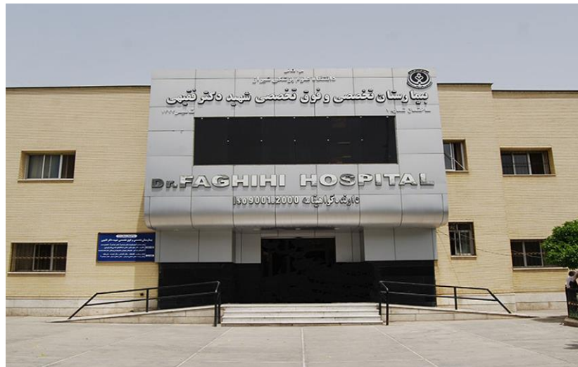
Figure 4: Faghihi Hospital Building, Source: Faghihi Hospital website, 1399
